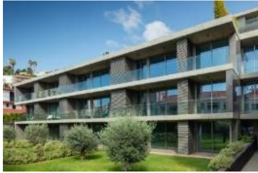
Fig. 28. Savoy Residence, RH+ Arquitectos, 2016, Casa Branca, Funchal, Madeira
