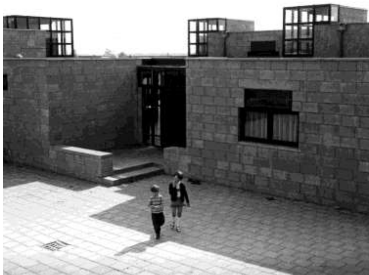
Figura 55-Entrada para a escola Montessori. Fonte: https://www.ahh.nl/index.php/en/projects2/9-onderwijs/114-montessori-school-delft
