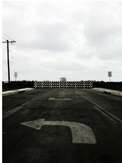
FIG. 4: Road infrastructure to accommodate future exurban development
