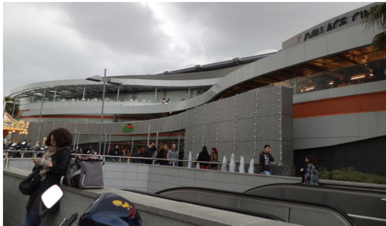
FIG 8: The entrance and the main façade of Athens Metro Mall (Photo courtesy of V. Tzani )
