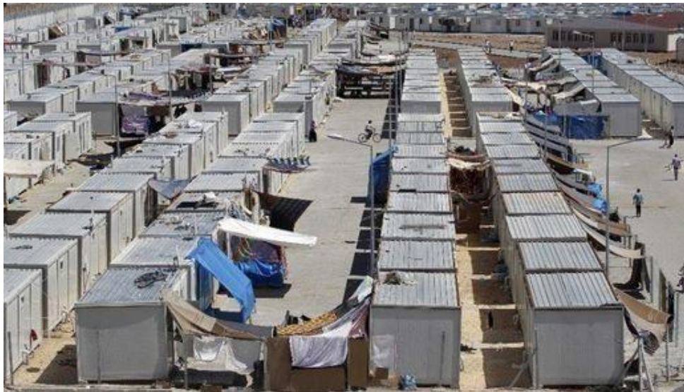
Figure 30. What refugees added to their containers: creating privacy and entrances with pieces of fabric, Zaatari camp, Jordan, 2013
