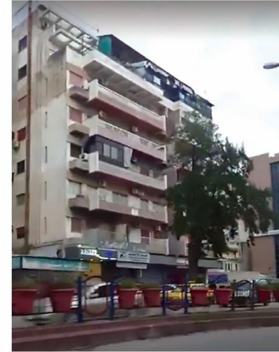
The Building on the site of the demolished Isrep mansion 2017, Rand Issa.
