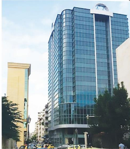
The Tower built on the site of the demolished Shidiaq mansion 2017, Rand Issa.
