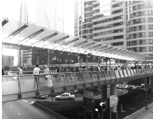
FIG 5. The Central Elevated Walkways over Connaught Road, Central, Hong Kong. Kwok, E October 2012
