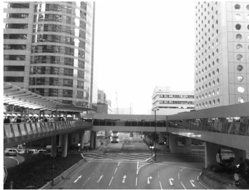
FIG 4. The Central Elevated Walkways over Connaught Road, Central, Hong Kong. Kwok, E October 2012
