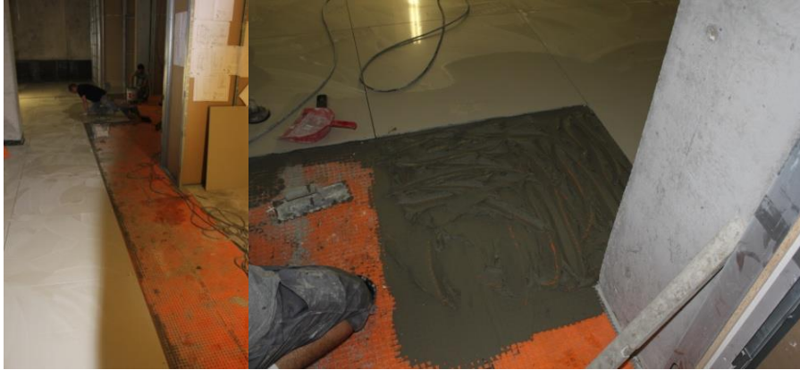
Figures 6 - 7 - The orange polyethylene Ditra membrane laid over the light concrete layer, the adhesive and the flooring tiles
