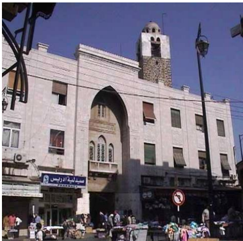
Fig. 53: The great mosque of Al-Nuri before destruction.
