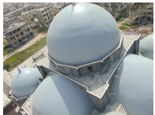
Fig. 59: The domes of Khalid Ibn Al-Walid mosque after reconstruction.
