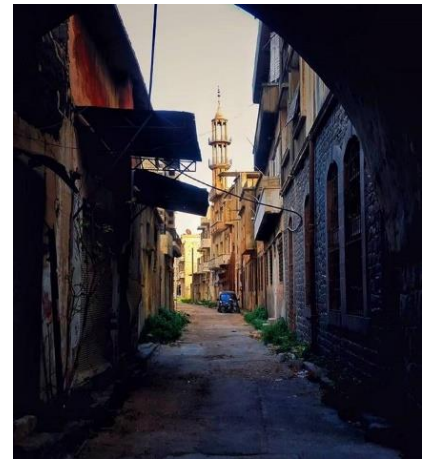
Fig.9: Al-hamidya neighbourhood, deterioration due to human activities.
