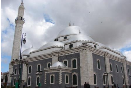
Fig.1: Khalid Ibn al-Walid Mosque-Homs, Syria. Before the destruction.
