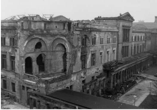
Fig. 32: The Neuse Museum after destruction, Berlin, Germany.
