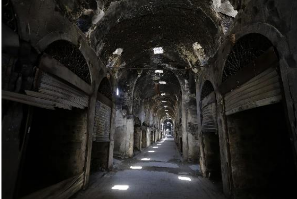
Fig. 49: The destruction in the covered market after the armed conflict.
