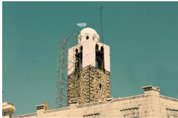
Fig. 55: Reconstruction works of the Minaret of the Great Mosque of Al-Nuri.
