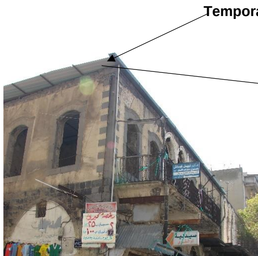
Fig. 73: Khan Al-Jamal, temporary roofing. (DGAM)
