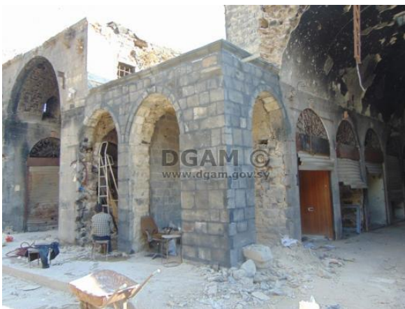
Fig.10: Ancient souk, Homs, Syria, deterioration due to political conditions
