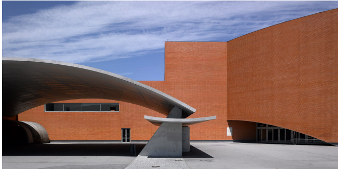
2. Pavilhão multi-usos, Gondomar
