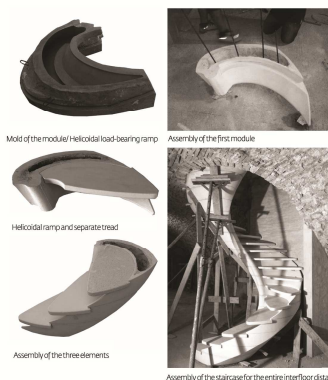
FIG.5. and 6. Prototype of the Re-composed Stair – version made of artificial stone with permanent formwork
