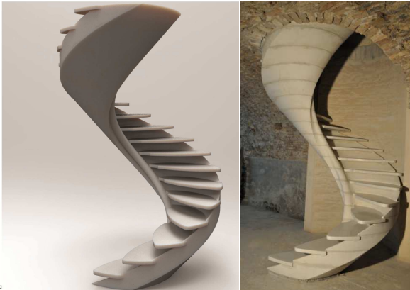
FIG.5. and 6. Prototype of the Re-composed Stair – version made of artificial stone with permanent formwork
