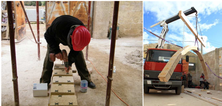
FIG.30. and 31. Flexible Arch Workshop
