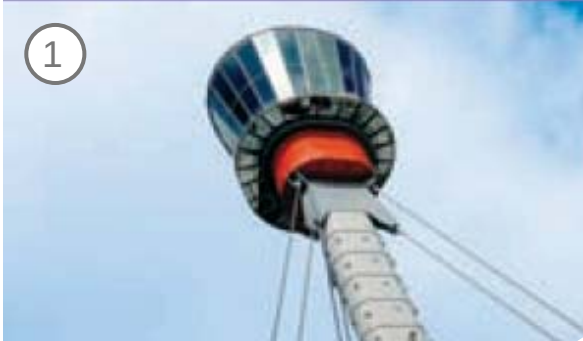
Air Traffic Control Tower
