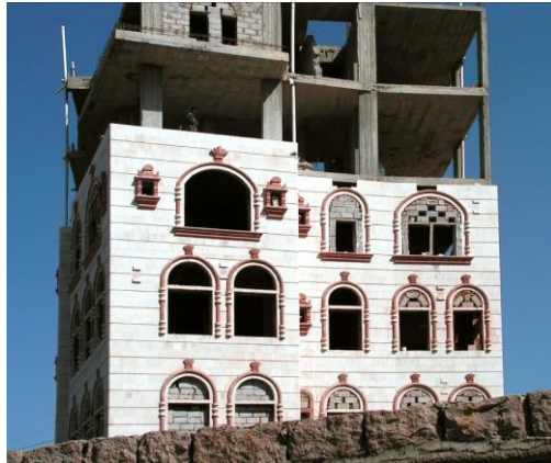
Fig 8. Al Habilayin. Mechanically cut stone making the façade of conventional concrete structures
