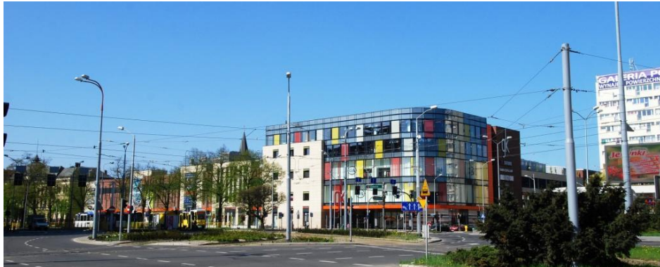
FIG. 9. Szczecin-Poland. The silhouette of the Galeria Kaskada shopping mall in the city context. Source: author
