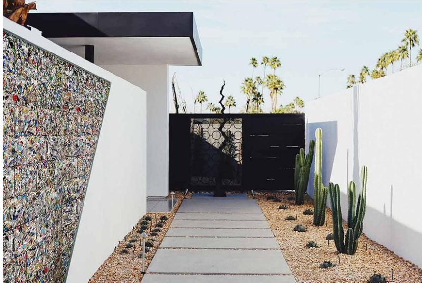
Figure 2.6 - Use of replast on a wall (ByFusion, 2023)
