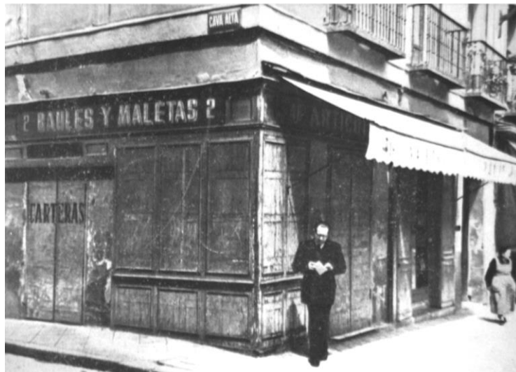
FIG. 1. Traditional store. 'Good wine needs no bush' (Photo: Revista Nacional de Arquitectura)
